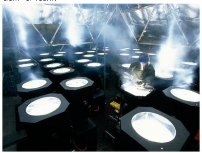
A technician handles one of 39 volatile 7,000-watt xenon lamps atop the Luxor pyramid on the Las Vegas Strip. Touted as the world's brightest light, Sky Beam is strong enough to read a book by—10 miles (16 kilometers) out in space.
