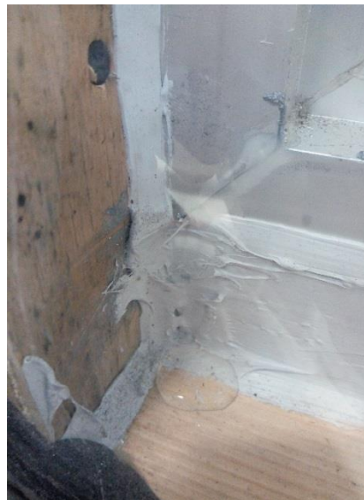
Photo No. 2 Leak observed from interior caulk joint
