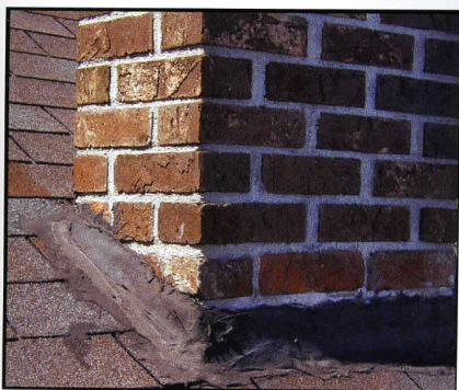
Chimney with cracked and deteriorated flashing
