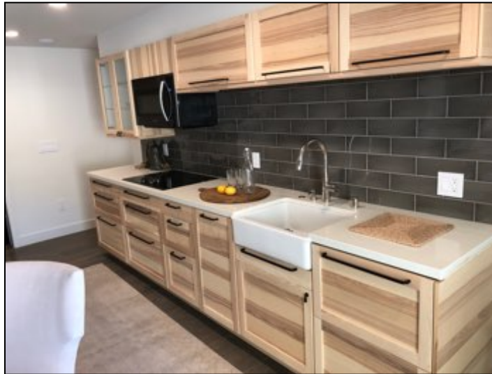
Kitchen Counters, cabinets, floor and lights appear in serviceable condition.
