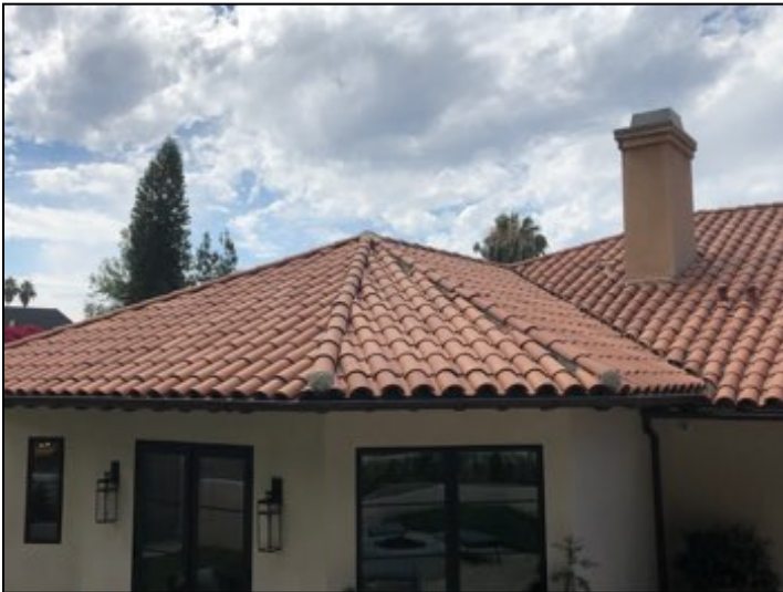
Main roof is clay tile, the majority of roof appears serviceable with few broken tiles. Recommend having broken roof tiles repaired as required to prevent moisture intrusion.
