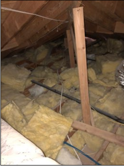
Insulation is fiberglass batts, approx 8" depth.
