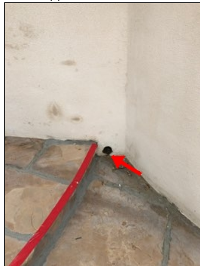
Visible drains at retaining walls, drains are not tested.
