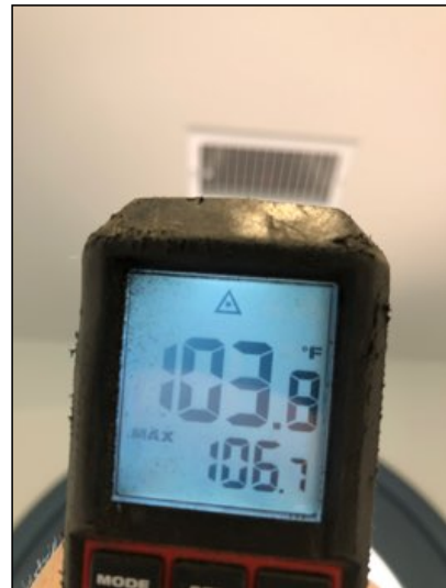
HVAC temperature on heating mode for Dining room is 103°F, appears serviceable.
