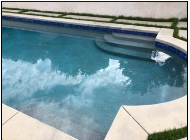
Pool plaster/plaster gunite appears serviceable.
