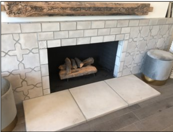
Fire place (A) located at family room.
