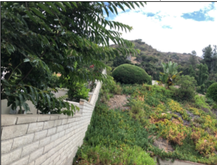
Fence at property is masonry block located on east side.
