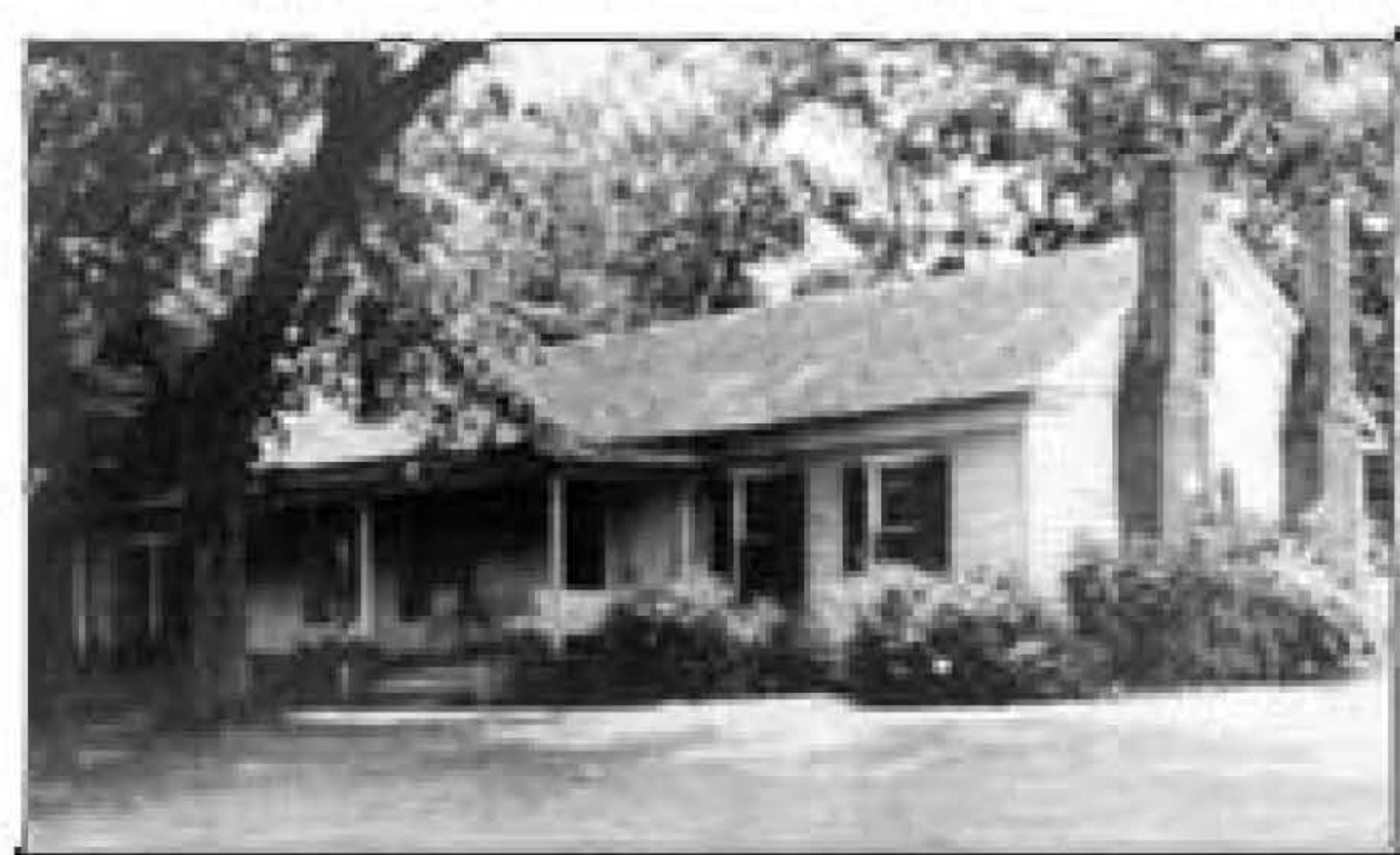
WILLIAM DICKINSON HOME Original home on site, 1840
